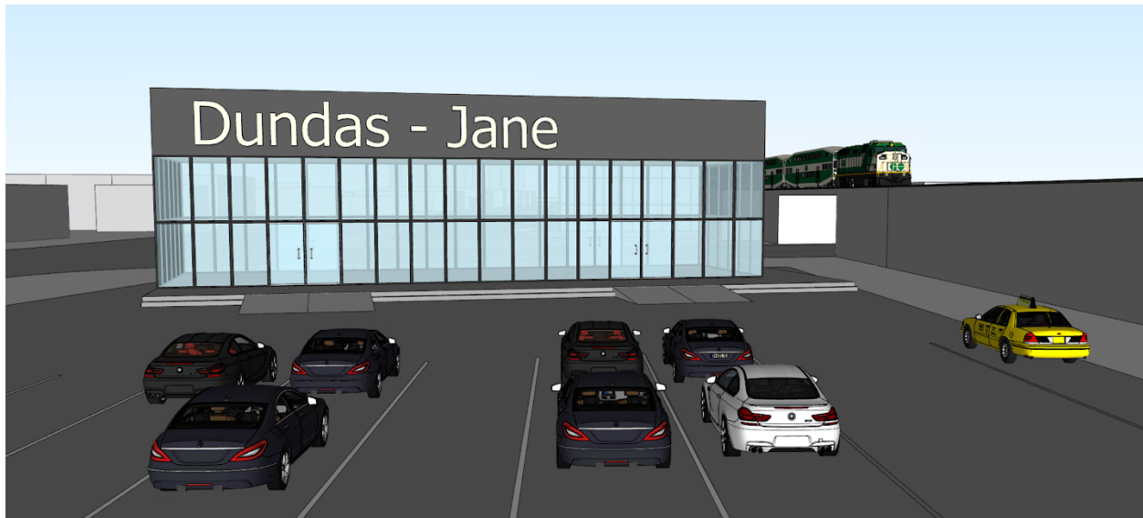
Figure 27: PPUDO and Secondary Station Building
